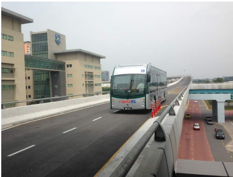
Figure 3: View from the SunU-Monash station showing Monash University and the electric bus used
