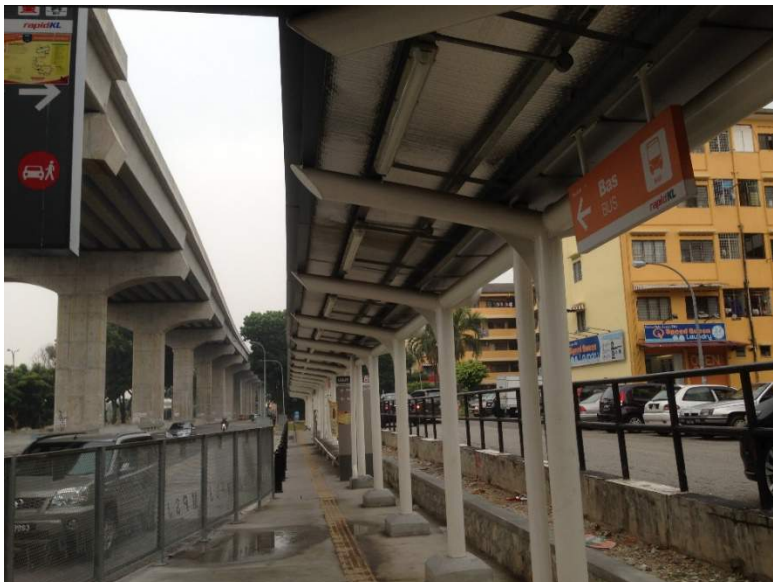
Figure 16 Featuring the short roof at the USJ7 bus laybys
